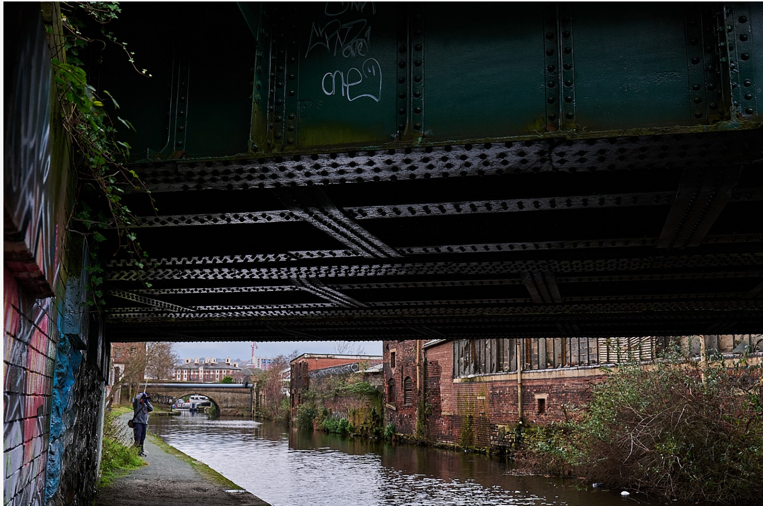
Under the bridge
