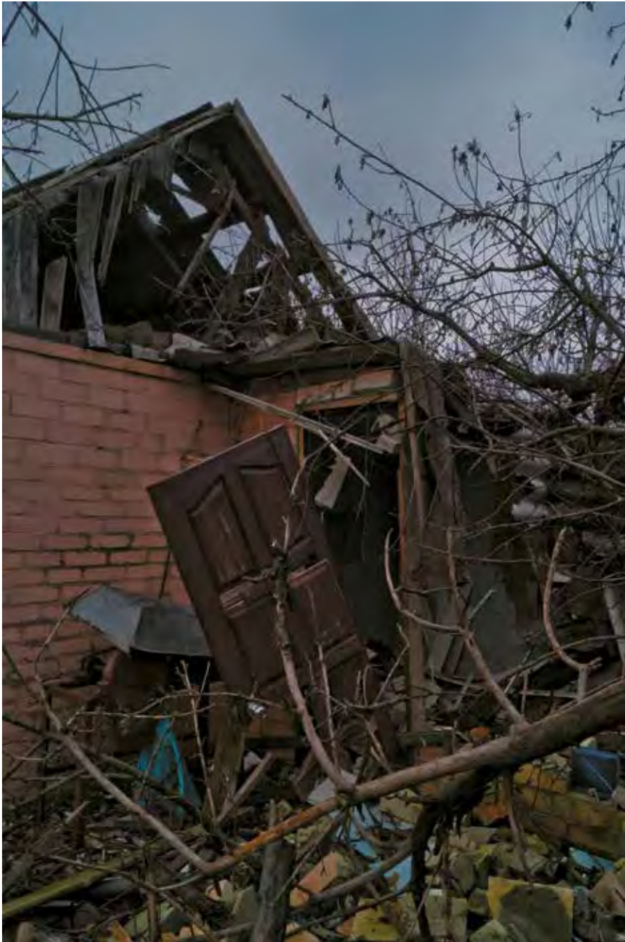
A ruined shed in our backyard. Cherkasy Tyshky
