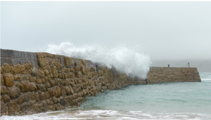
Above and overleaf Sennen Cove sea wall and beach
